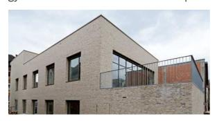
In 2015 the first municipal low-energy building, a canteen including a small gym on the campus of a school centre, could open in Ludwigsburg, thanks to funding received under the EU project "CEC5". With its very good insulation the compact building fulfills the energy standards of a passive house.
